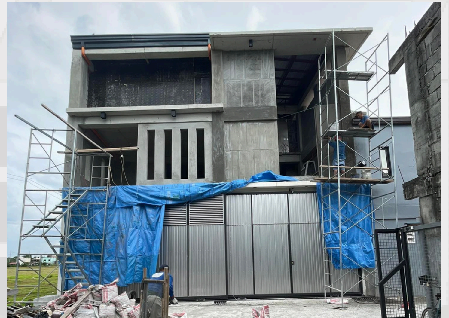
Site Progress as of February 2023
